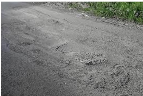
Figure 5: The above diagram shows the disintegration, which results as a loss of bonding, chemical reactivity etc because to the lack of materials [fineartamerica].
