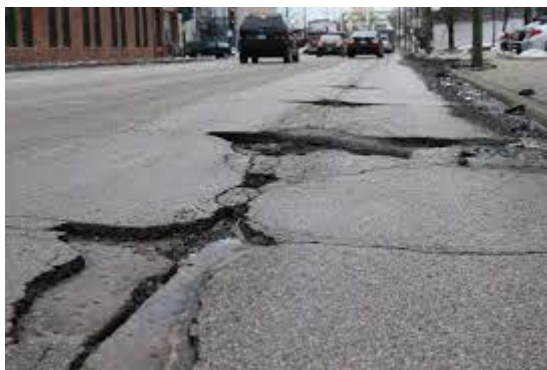
Figure 3: The above diagram shows the fracture, which are made by the large vehicle travelling with the large amount of loads. [mediaindia].
